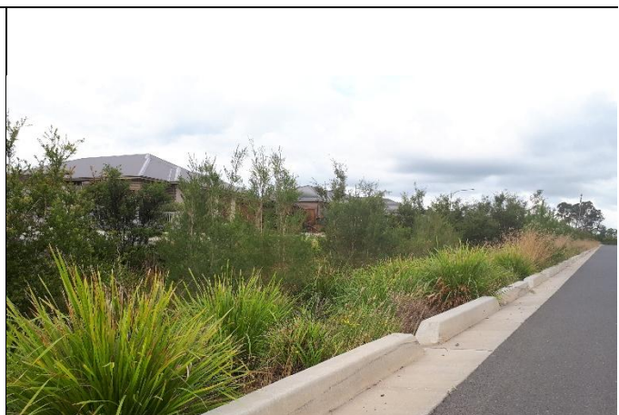
Central median swale with trees (The Oaks, Wollondilly Shire Council). Source: Wave Consulting Australia.
