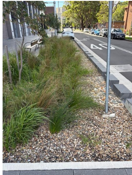
Bioswale alongside street (long view), with rock inlet to manage scouring (Redfern, City of Sydney). Source: Wollondilly Shire Council.
