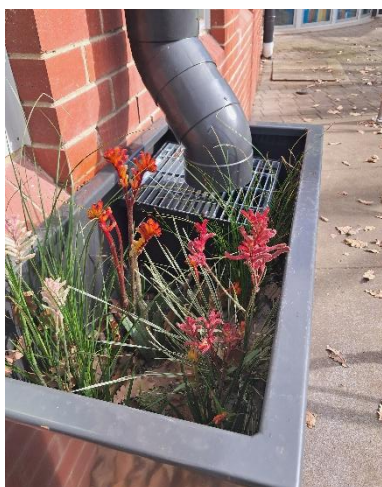
Above ground raingarden (aka WSUD Planter box). (Coburg, Merri-bek City Council). Note – local native species like viola hederacea would be more suitable for these systems in Wollondilly Council. Source: Aqua Build Manufacturing.
