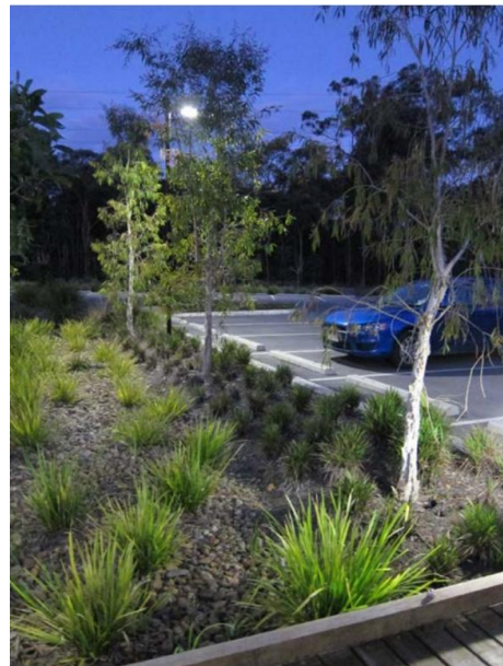
Swale adjacent to car park (Logan City Council) Source: Water by Design, Jack Mullaly.
