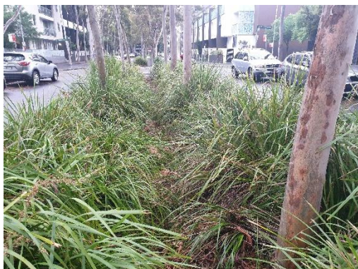
Central median swale with trees (Zetland, City of Sydney). Source: Wave Consulting Australia.
