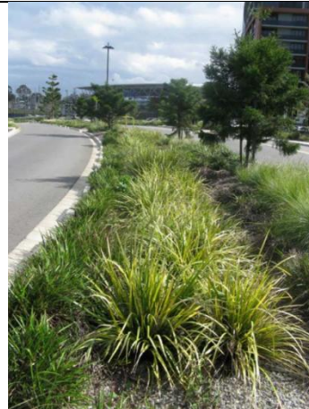
Central median swale with cascated kerbs (City of Sydney). Source: Wave Consulting Australia.
