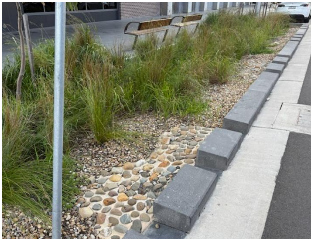
Bioswale alongside street, with rock inlet to manage scouring (Redfern, City of Sydney). Source: Wollondilly Shire Council.
