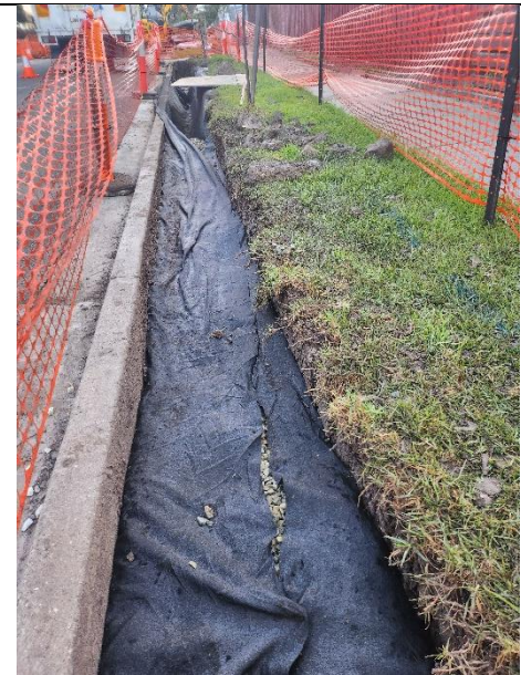
Infiltration trench prior to top soil, with geofabric wrap. Note other liner and aggie not shown after the back filling is complete. Source: Wave Consulting Australia.
