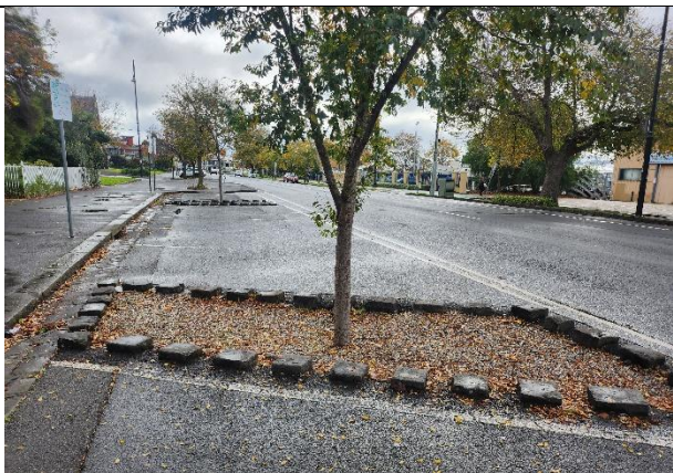
Tree pit installation with no ground cover. Castellated kerb used to allow multiple water inlets. This asset could benefit from increased ground cover to reduce urban heat, and increase evapotranspiration. (City of Hobsons Bay) Source: Wave Consulting Australia.
