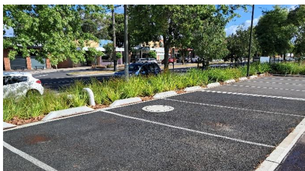
Raingarden installed in nature strip (Malvern East, City of Stonnington). Source: Wave Consulting Australia.
