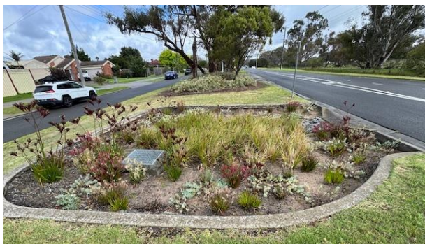
Raingarden installed in dividing strip (City of Kingston). Source: Wave Consulting Australia.
