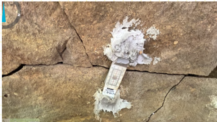
crack monitor showing no movement
