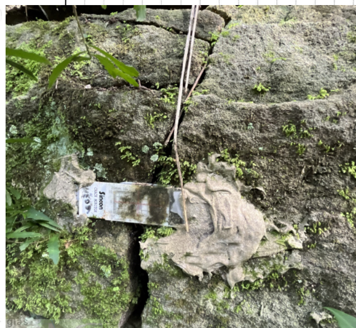
crack monitor on block on "new" wall
