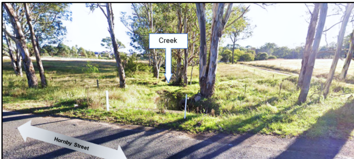
View from Hornby Street - Stringybark creek flowing from north passing under Hornby Street
